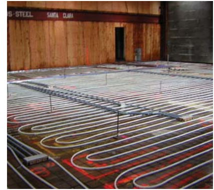
IDeAs offices in San Jose, California. Shown above are main entry, building integrated photovoltaic system with skylights, and PEX tubing for radiant floor during installation. Images courtesy of IDeAs
