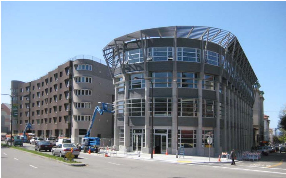
Contractors completing the David Brower Center (building at right) earlier this year.
