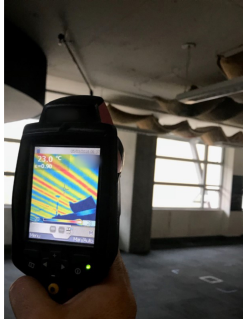
Infrared picture of ceiling with high-thermal mass radiant system.
