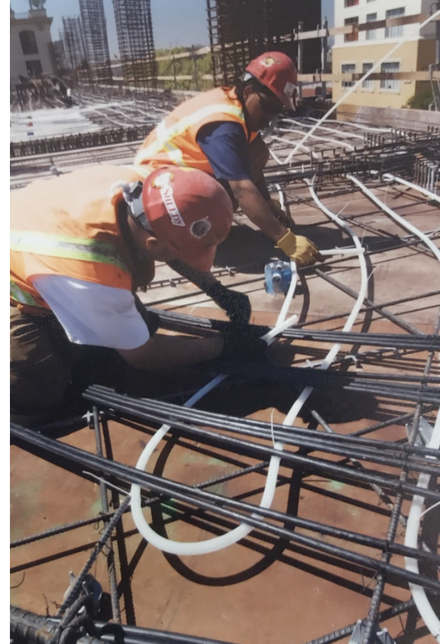
Construction workers installing high thermal mass radiant system.
