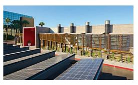
to generate the 135,000 kilowatthours (kWh) of estimated total annual building electrical usage. During its first year in operation, it actually exceeded that goal and generated more than 140,000 kWh of electricity.
