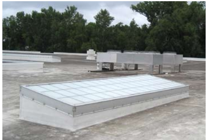
Skylights provide daylight where needed
