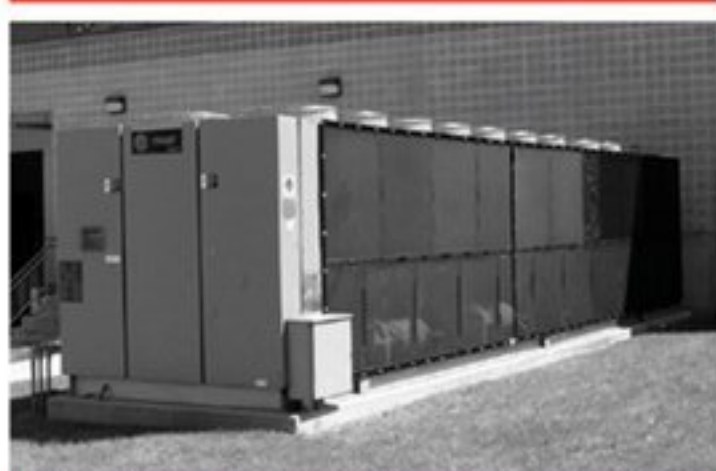
Air Cooled Chiller and Condensing Unit Filters
