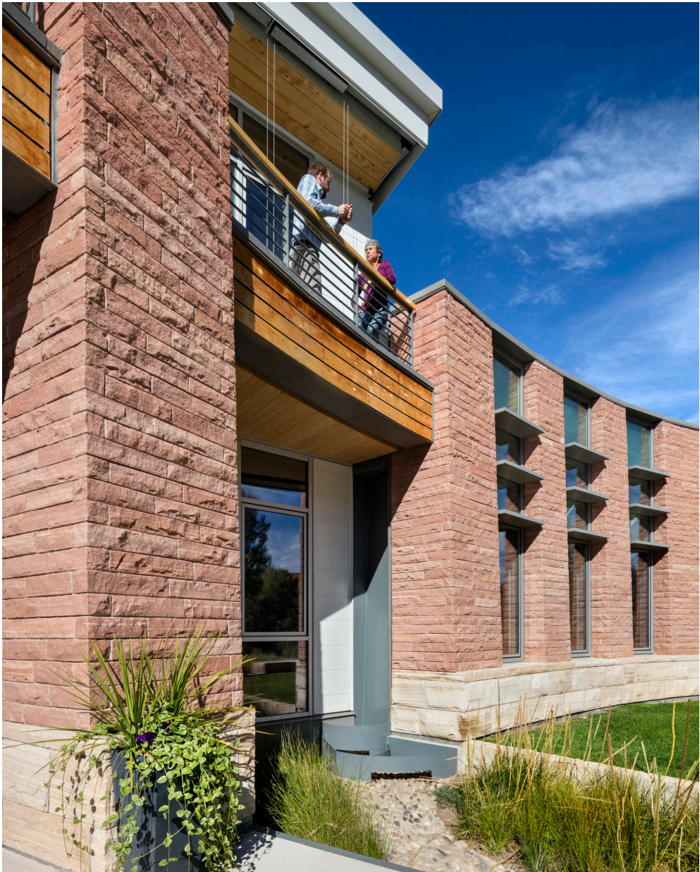
RIGHT During rain and snowmelt, the 7,700 SF roof captures, collects and directs water to a vertical water structure for future reuse.
