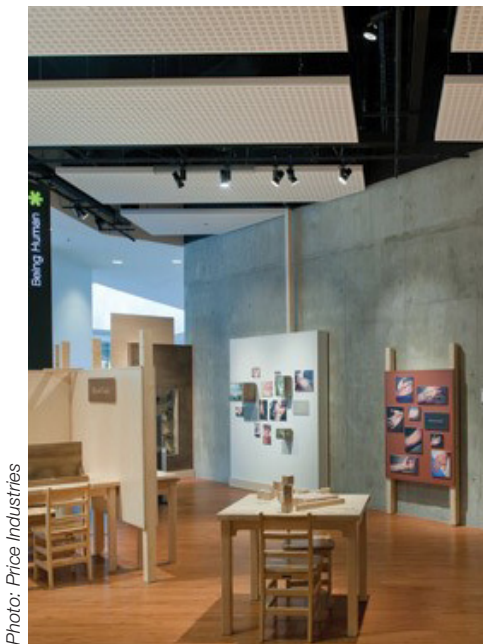
TELUS Spark Radiant Ceiling Panels
