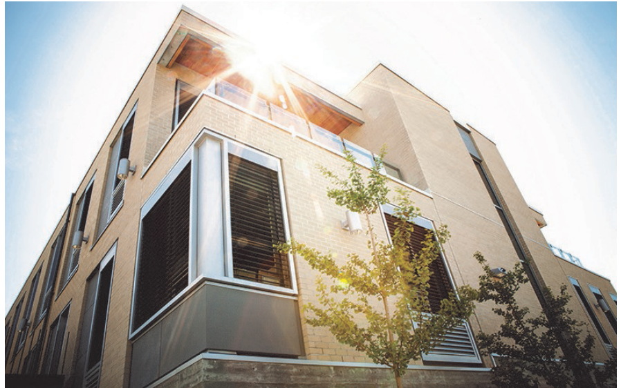
Trickle vents for passive ventilation. Photo: Reliable Controls
