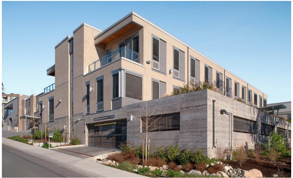
Photo: D'Ambrosio Architecture + Urbanism
