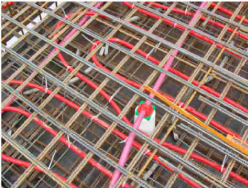
reinforced concrete slab with heating and cooling pipes - before pouring the concrete
