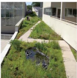
Green roof creates 30% or greater runoff reduction vs standard roof
