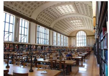
Wireless controls from Acura will control lighting in Doe Library’s main reading room.
