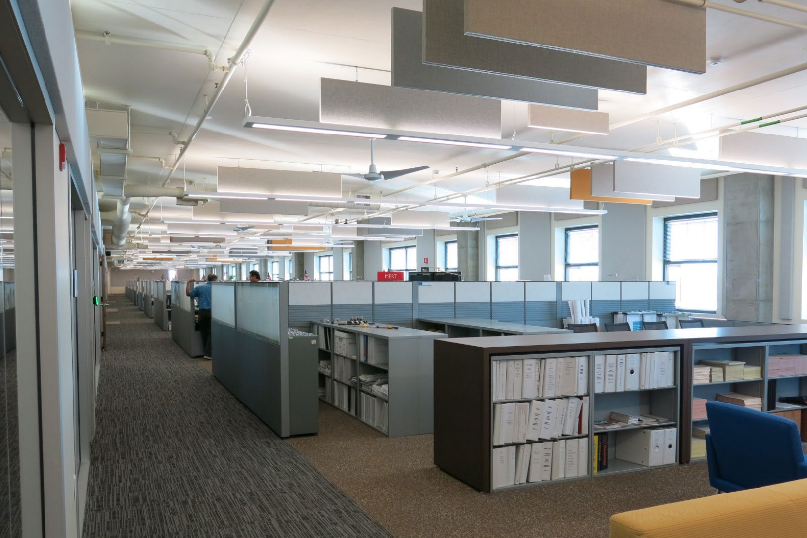
Open plan areas in SMUD's ZNE operations center feature exposed radiant ceiling slabs, vertically suspended acoustical panels, and ceiling fans. Photos: Caroline Karmann.
