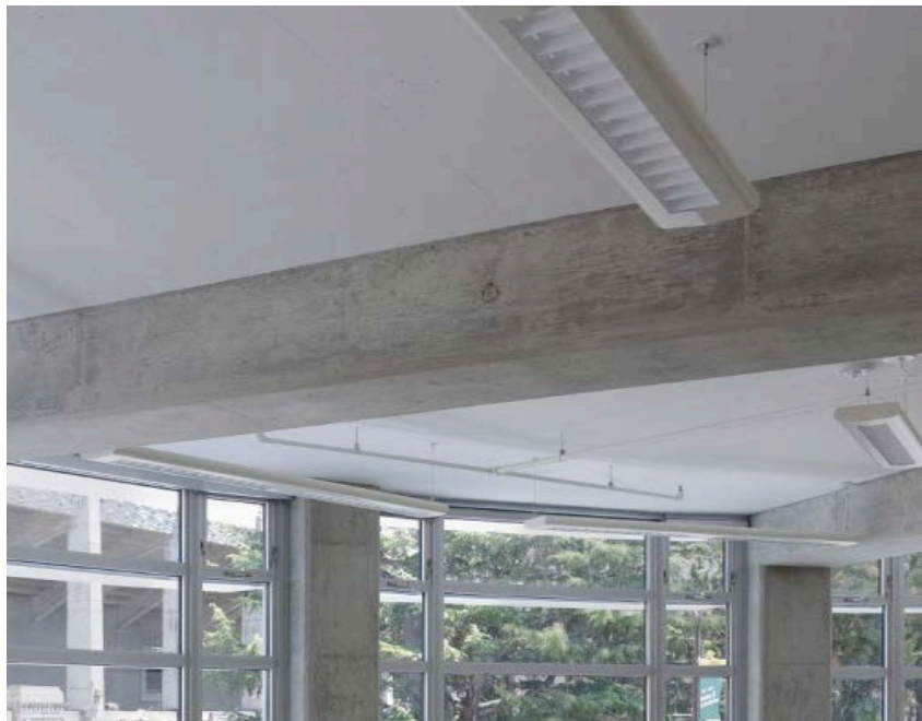
Concrete ceiling (Brower Center) Image: Tom Griffith
