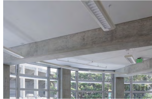
Concrete ceiling (Brower Center) Image: Tom Griffith
