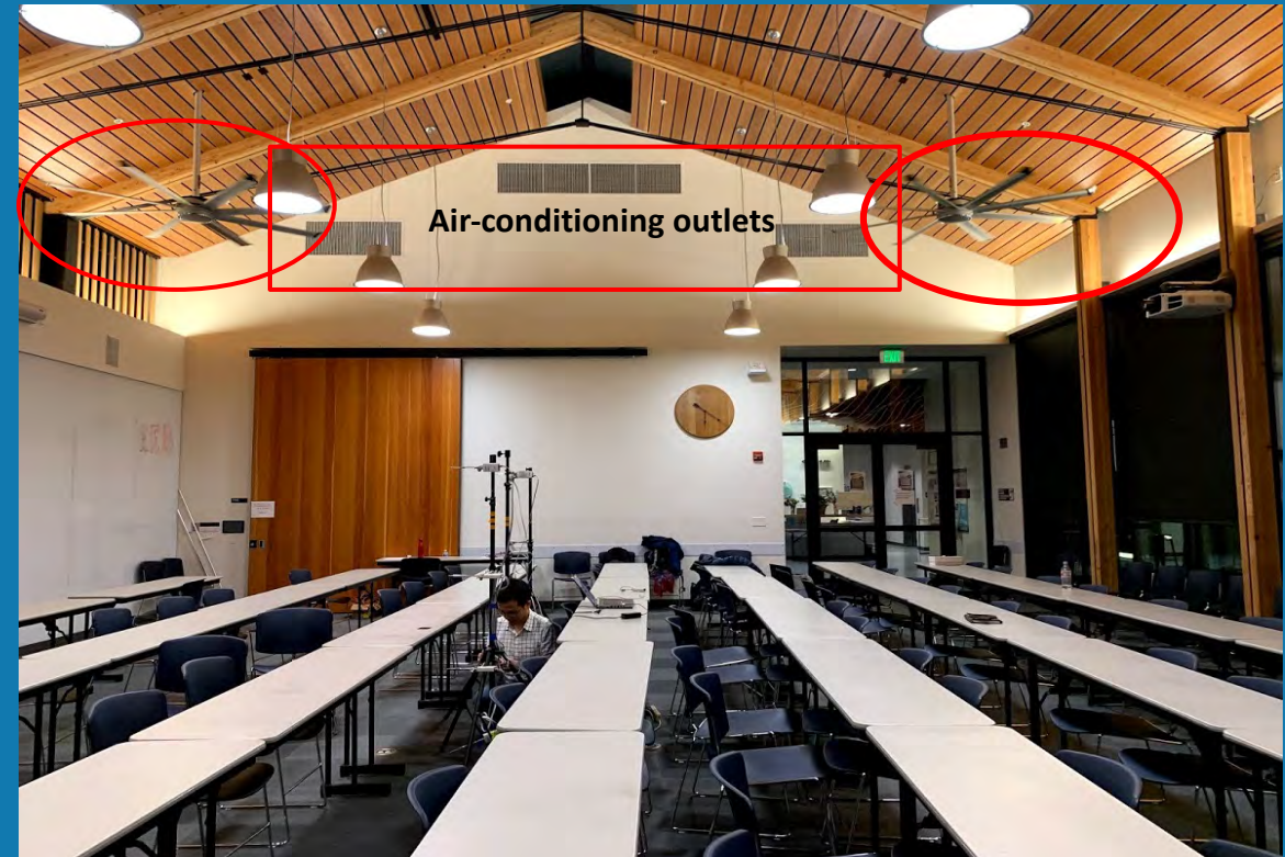
Santa Cruz biology seminar room, HVAC designed by Taylor Engineering
