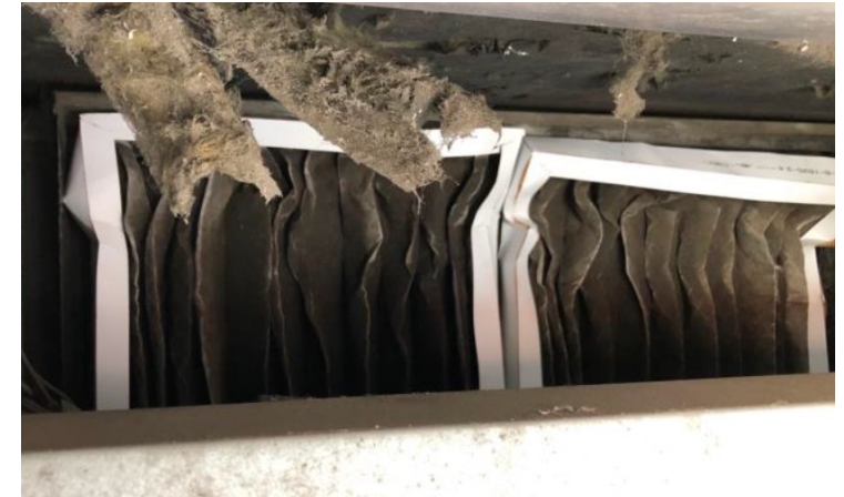
Dirty and crushed air filters
