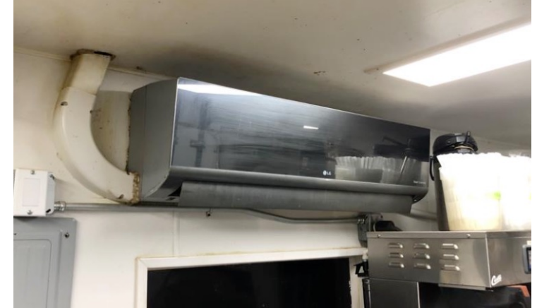
Undersized ductless split system air handler
