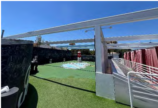
Steel- Reuse for Rooftop Garden
