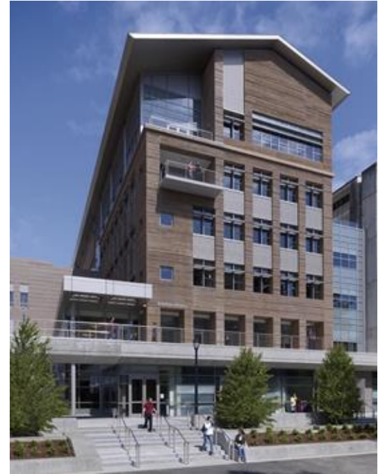
(Case study building)
